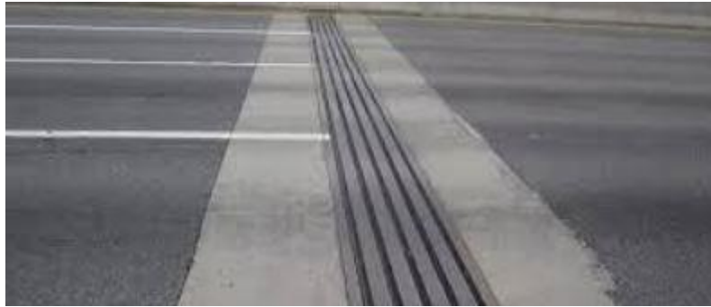
Figure 2.11 Typical modular joint (Mayer)
