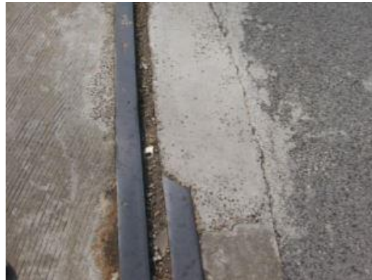
Figure 2.9 Compression joint with broken anchor (Miller)
