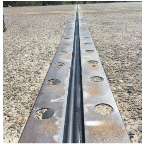
Figure 2.7 EMSEAL BEJS retrofit (EMSEAL)
