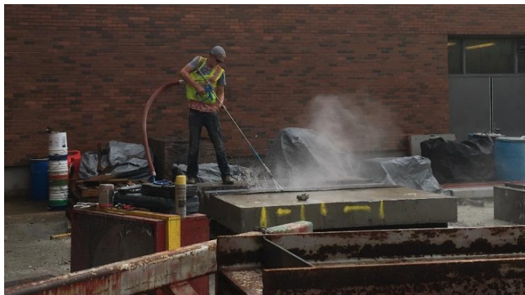
Figure 5.13 Cleaning the joint after hydrodemolition (Ruble)
