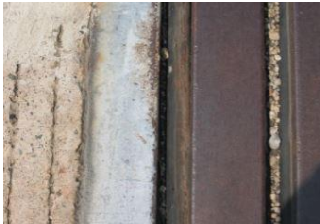
Figure 2.12 Modular joint with debris, preventing closure (Miller)
