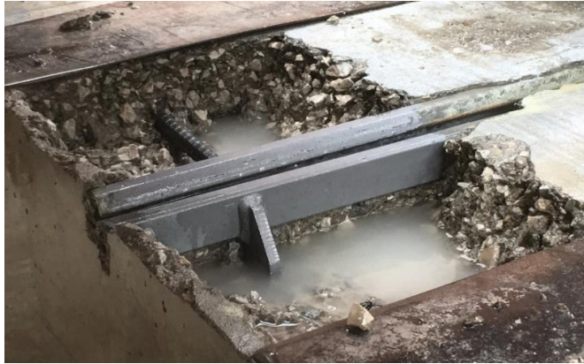
Figure 5.12 Hydrodemolition progress (Ruble)
