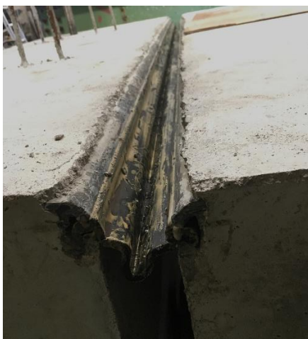
Figure 5.1 D.S. Brown A2R-400 strip seal (Ruble)
