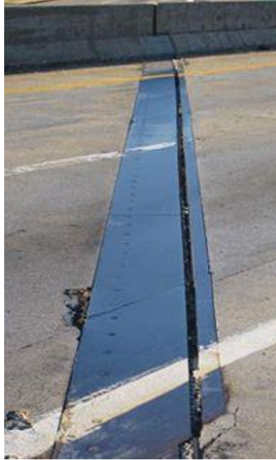
Figure 2.1 Typical sliding plate joint (MO DOT)
