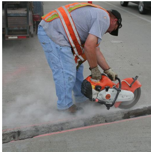
Figure 2.13 Saw cutting (EMSEAL)
