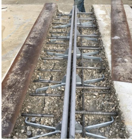
Figure 5.14 Completed hydrodemolition (Ruble)
