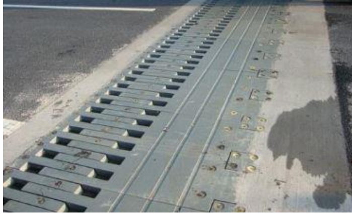
Figure 2.10 Typical finger joint (Haider)
