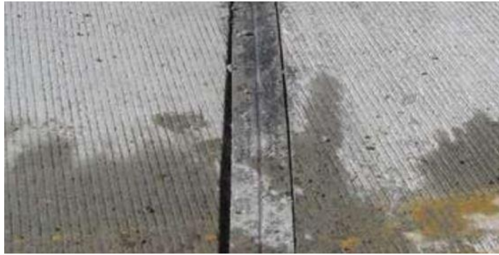
Figure 2.8 Typical compression joint (MO DOT)
