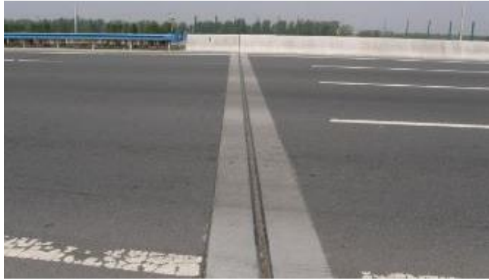
Figure 2.4 Typical strip seal joint (ArchiExpo)
