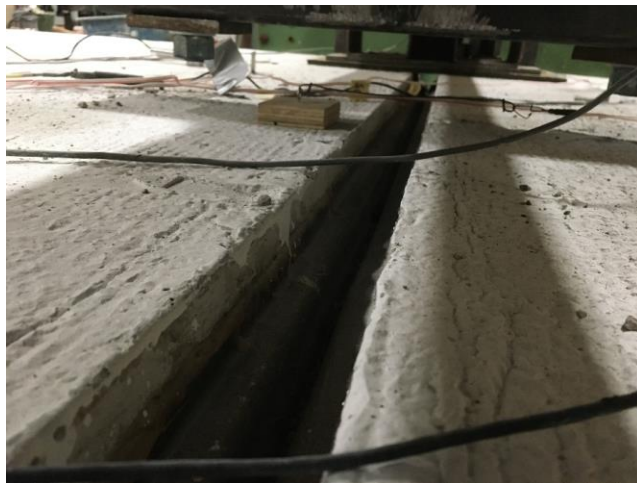
Figure 5.31 Visual inspection of joint (Ruble)
